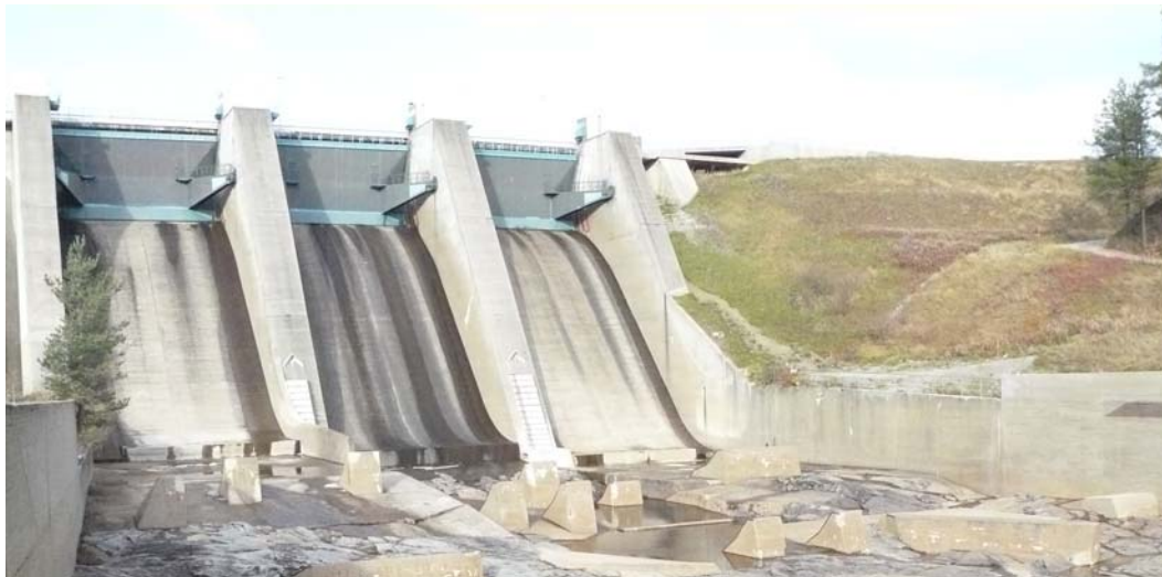
Figure 6.1 Photo of the spillway at Långbjörn concrete dam. The monolith for column 3, analysed in this chapter, is the second one from the right side in the picture.
