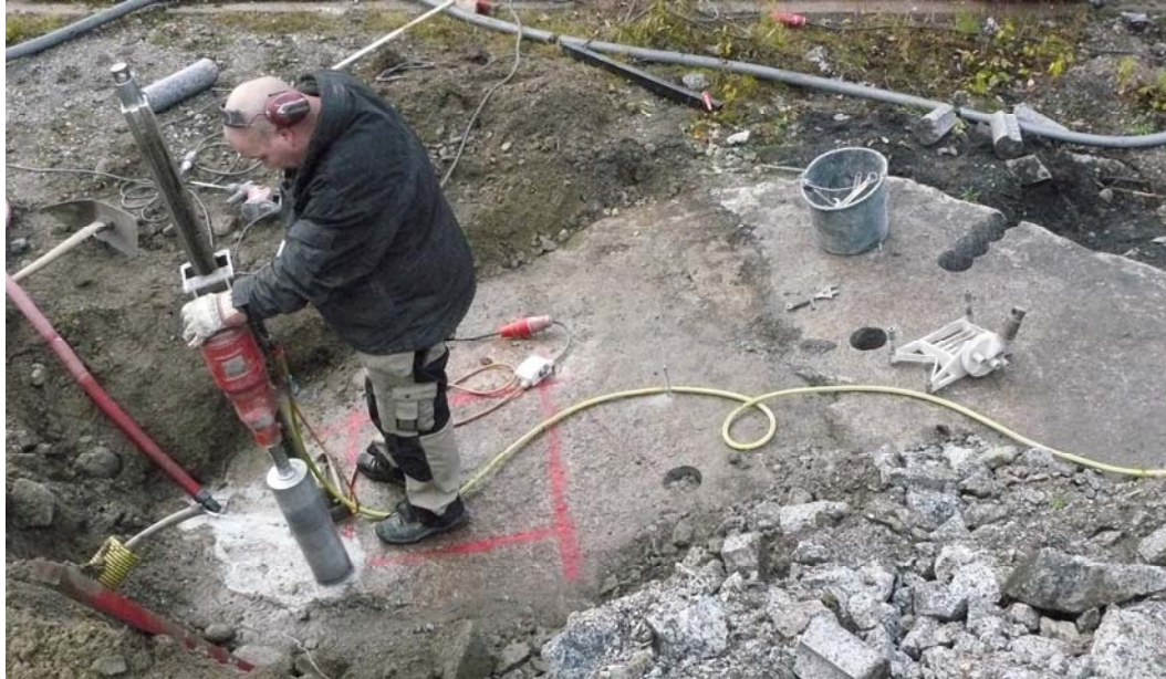
Figure 5.25 Drilling of vertical cores in order to investigate the extent and inclination of the assumed location of the persistent joint.
