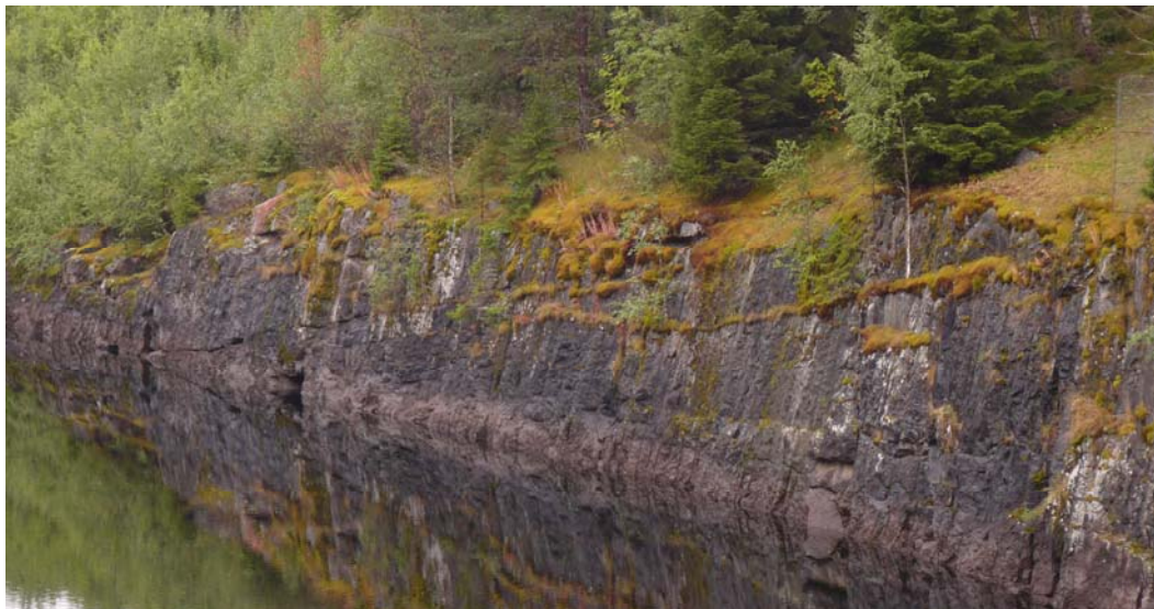
Figure 5.2 Photo of persistent relaxation joints in the tailrace channel.
