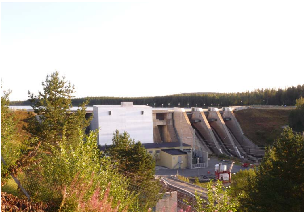
Figure 5.1 Overview of Långbjörn hydropower station.
