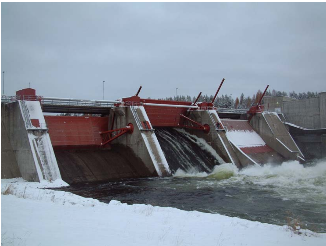
Figure 1.1 Spillway of the concrete dam at Pengfors hydroelectric power station, one of many in Sweden (Photo: SWECO VBB).
