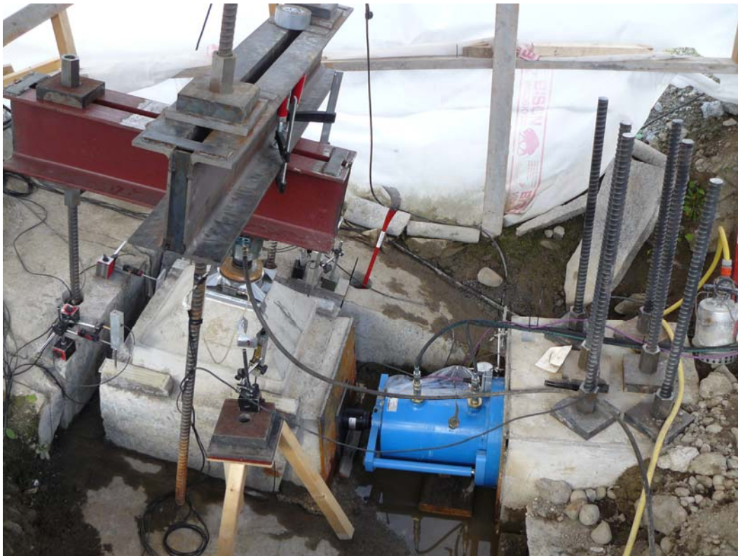
Figure 5.27 Photo of the test site during the shear test.
