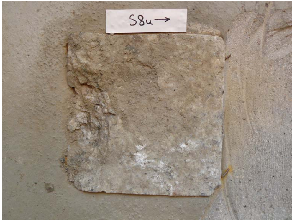
Picture B.7a Sample S8 after the shear test (lower part).
